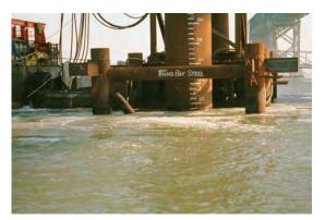
Figure 3-9. Air bubble curtain in operation. Source: Caltrans (2001)
